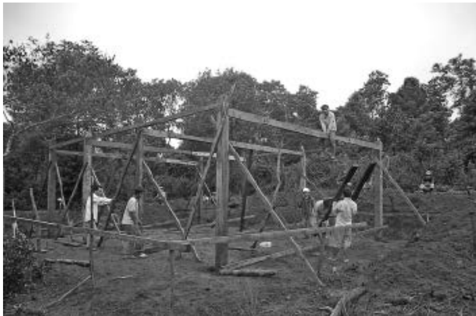
Mobile skills training on a site
